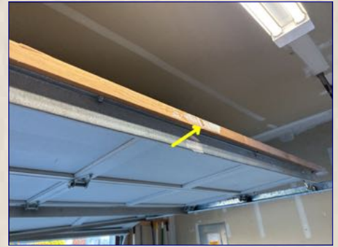
Recommend painting the outside edges to help prevent water damage.
