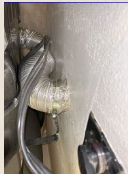
The dryer vent connection.
