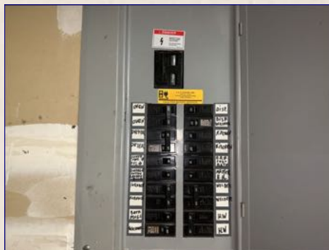
The main electrical service panel
