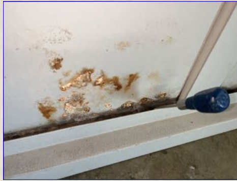
The lower panel of the overhead door had significant water damage. Replacement of the panel by a qualified professional is recommended.
