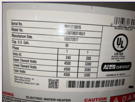
The Water Heater Data Tag
