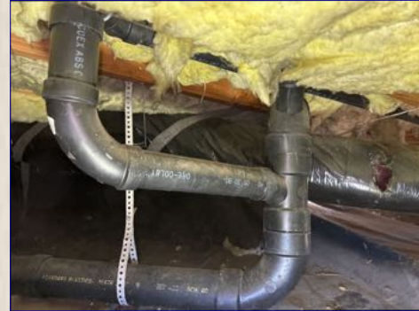
The visible drain/waste piping
