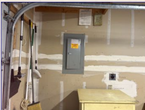
The main electrical service panel
