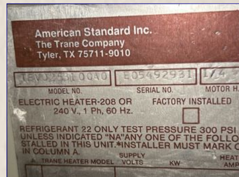
The furnace data plate
