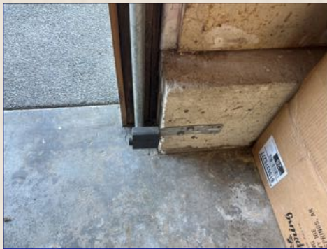
The electric eyes on the garage door opener had been bypassed. This is a safety hazard. Repair by a qualified professional is recommended.
