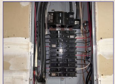
The main electrical service panel
